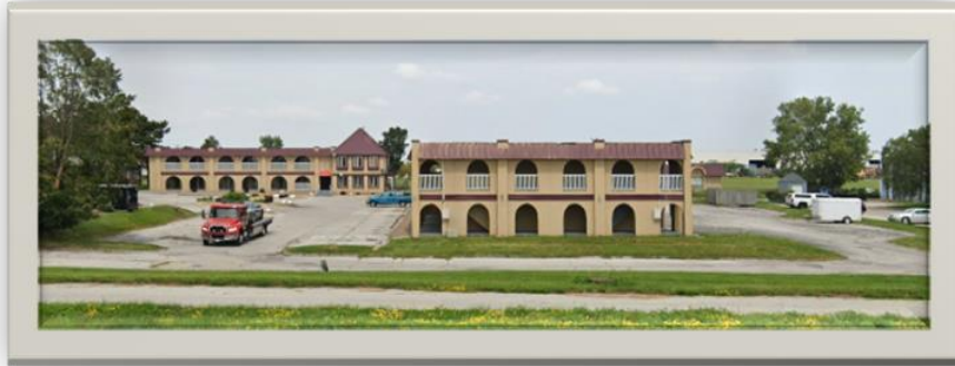
Before Acquisition and Demolition
