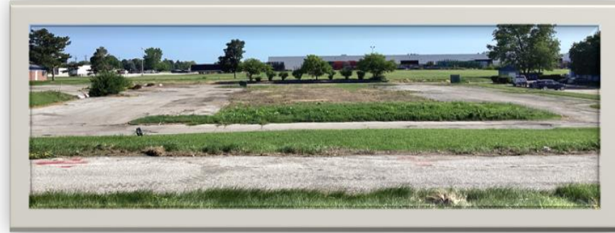
After Demolition, Investment Ready
